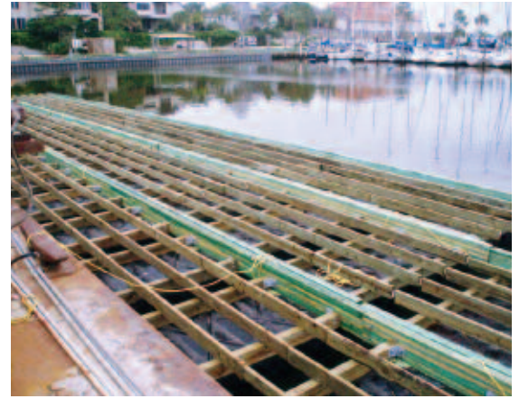
Treated glulams supporting floating dock
