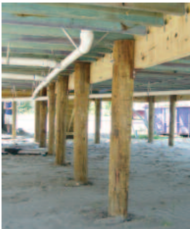
Round timber piling
