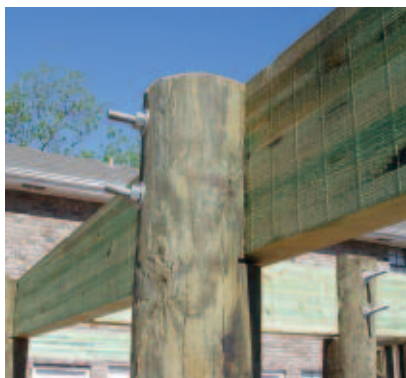
Pressure-treated glulam beam
