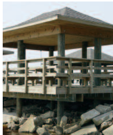
Round timber piling – marine application
