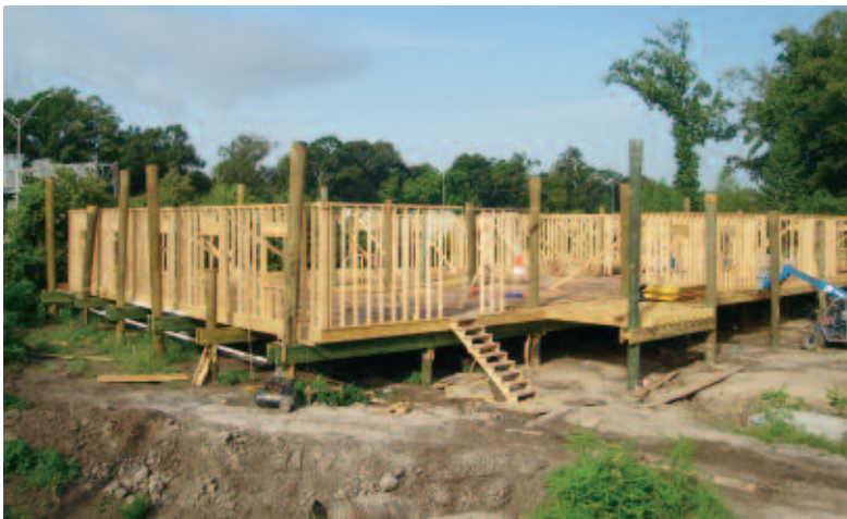
Round Timber piling and glulam floor beams
