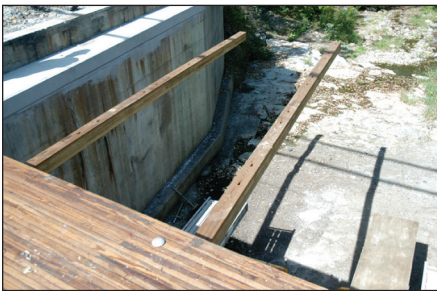
Figure 3.6. Longitudinal glulam deck stiffener details.
