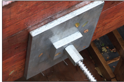
Figure 3.13. Stress-laminated glulam deck stressing detail.
