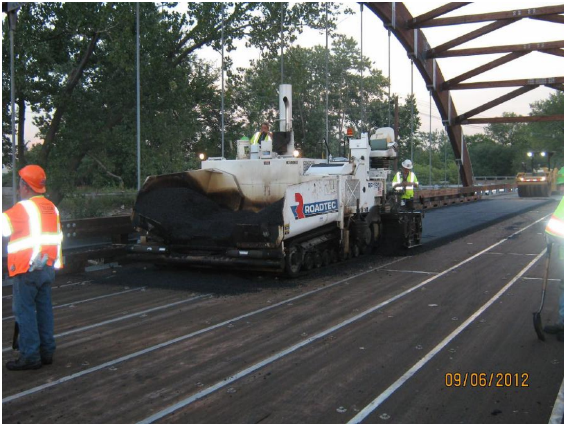
Photo 5. Paving operations on the Overpeck Park Bridges
