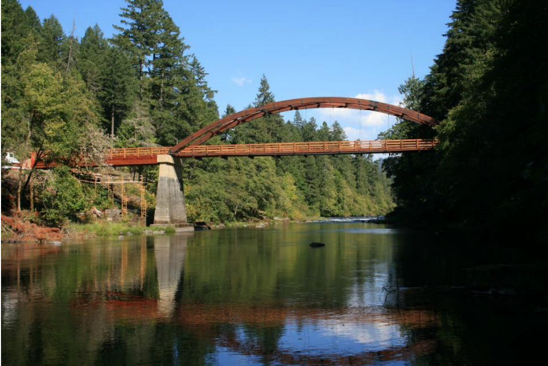
Photo 7. Tioga Bridge over the North Umpqua River
