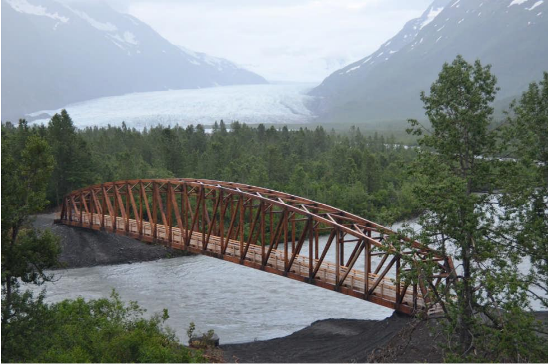
Photo 3. The Whistle Stop Bridge in Portage Alaska (Photo courtesy of Eleanor Oman, US Forest Service)
